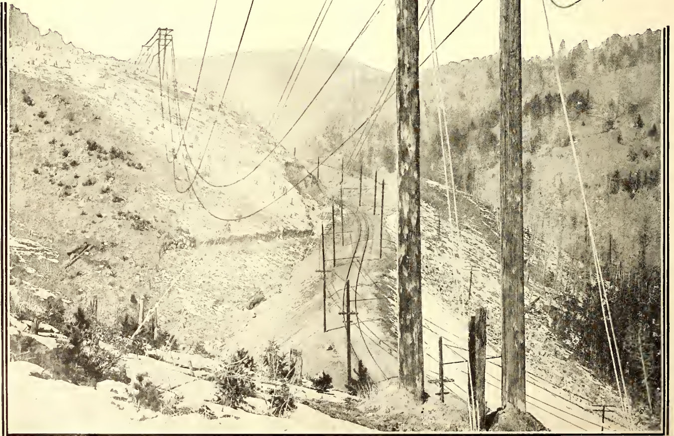
On Chicago, Milwaukee & St. Paul Railway, 20 miles east of Butte, Montana. Weight supported by Pole Structure in foreground, 1335 pounds. Height of Pole above ground, 30 ft.; length of Span, 970 ft.
